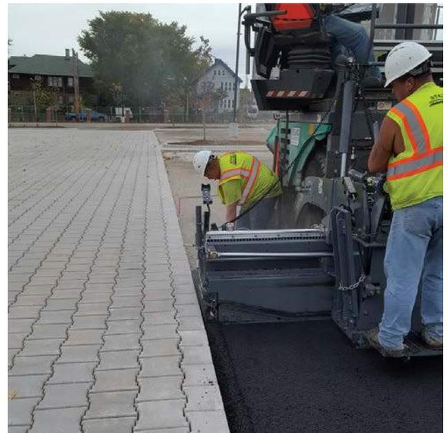
PaveDrain blocks work with existing infrastructure and can be used as the form for concrete or asphalt pours. Half blocks and end blocks square off corners eliminating cutting AND small pieces that are easier to dislodge.
