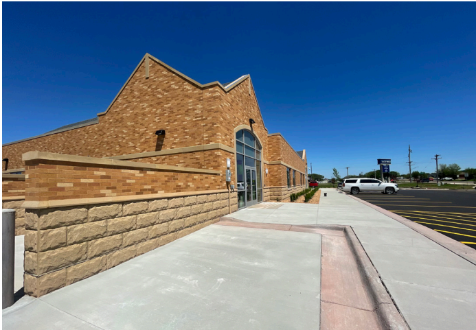
Sanford Clinic: Stone Mason Unit (Limerock)
