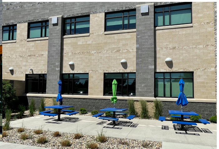
Capital Services: Burnished Unit (Onyx and Nutmeg) Travertina Unit - (Onyx and Nutmeg) Rock Face Unit - (Onyx)
